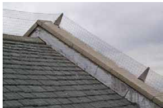
Bird Netting on roof eave
