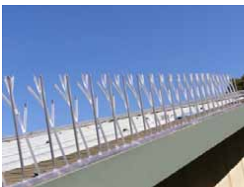
Bird Spikes on roof eave
